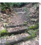
Inset logs steps with treads cut into the log, which are showing evidence of age and decay. Do not meet code for slip resistant. Native soil surface is subject to erosion, even with the existing Wood-Water Bars.
