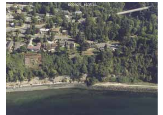
View of disconnected feeder bluff in park (right) and connected feeder bluff adjacent to park (left)
