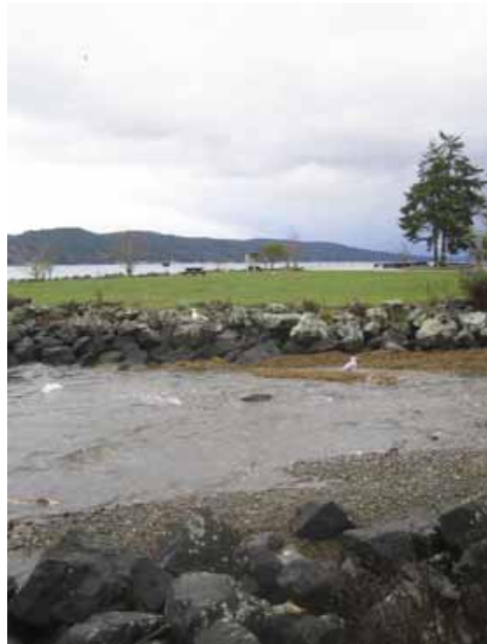
Armored creek mouth with narrow band of marsh vegetation. Note: armored boat ramp extending far into intertidal zone.
