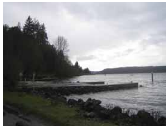
Boat ramp with solid concrete foundation that prevents longshore sediment movement
