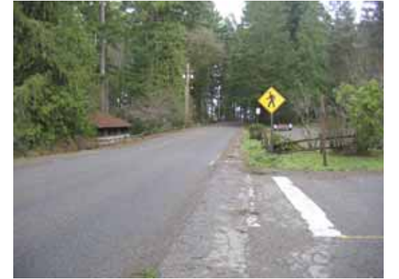
State route 106 runs along the south shore of the Hood Canal and bisects the park
