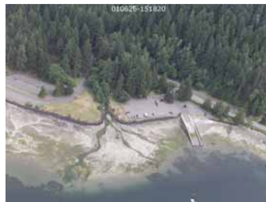
Armored mouth of Twanoh Creek and Puget Sound Shoreline
