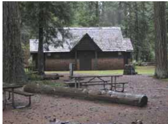
Campground south of Highway 106
