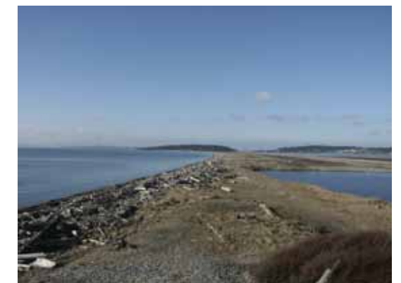
View of spit and low elevation of Highway 20
