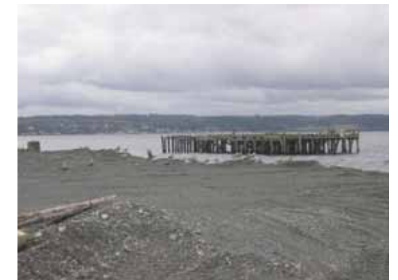
Existing Quartermaster wharf structure
