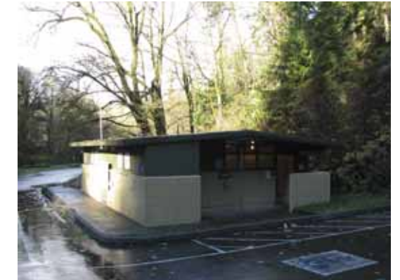
Existing comfort station at Saltwater State Park
