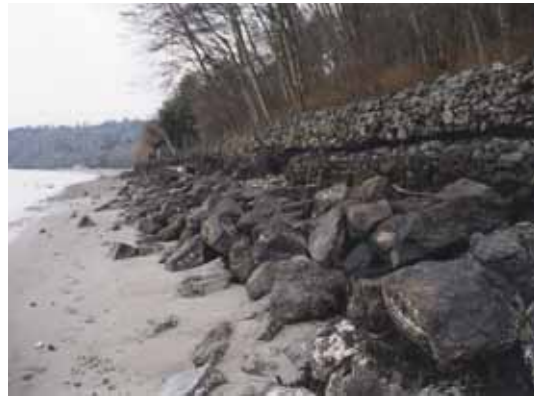
Example of a shoreline armored with rip rap
