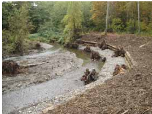
Example of meandering stream and constructed logjam for habitat at higher flows
