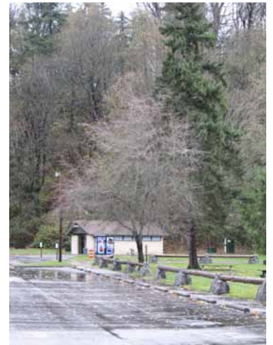
Existing comfort station and parking lot near the shoreline at Saltwater State Park.
