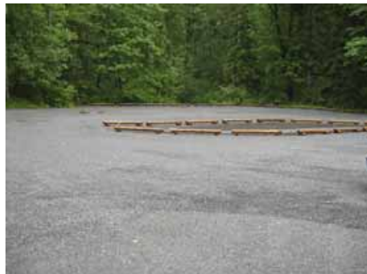
Gravel parking with stormwater treatment in the center
