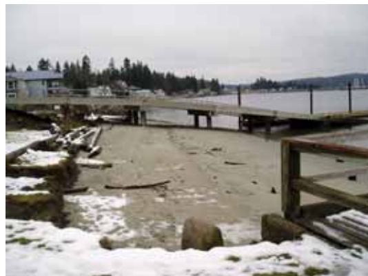
Example of bridged boat ramp to prevent interruption of sediment transport. Source: D. Small, WDFW
