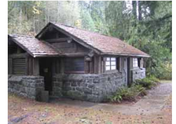
Existing comfort station at Twanoh
