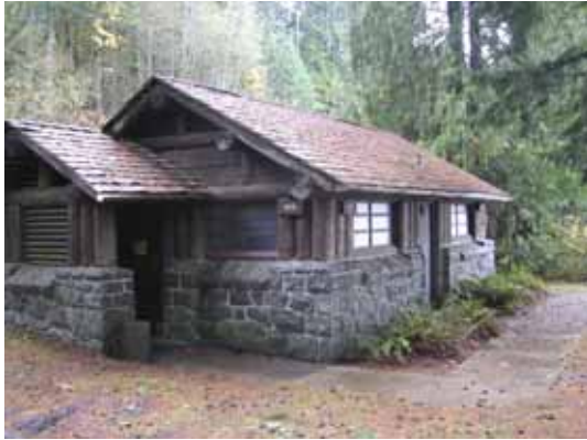
Existing buildings, like this restroom, can be maintained sustainably
