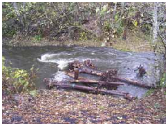
Added large woody debris in stream
