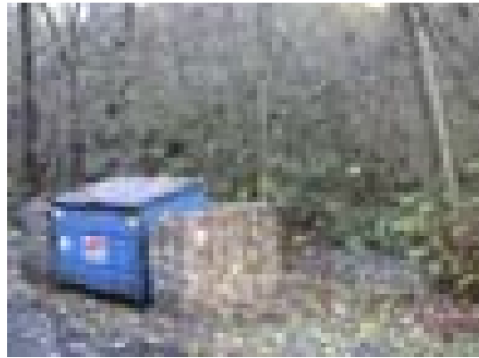
The existing trash area enclosure next to McSorley Creek could be relocated outside of the riparian corridor.
