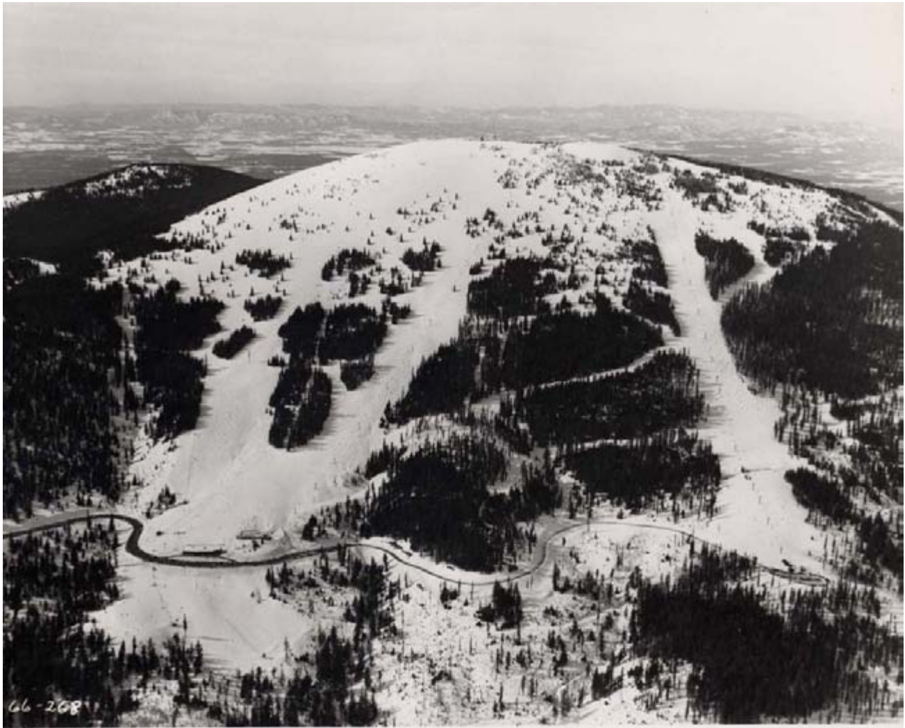
Looking west at the east slope ski facilities on Mount Spokane. This photograph was taken prior to construction of Lodge #2 (WSPRC).
